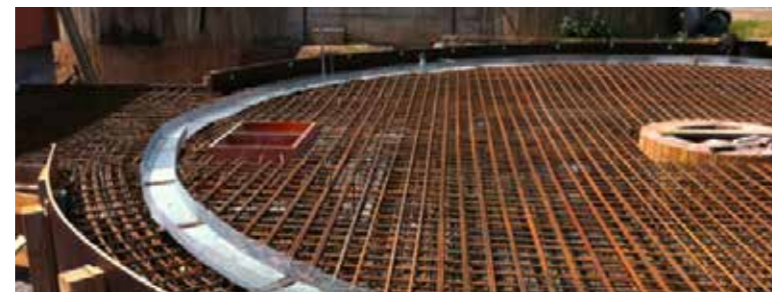
Shuttering System for Vessel construction
