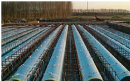
Used as „hollow blocks“ in order to reduce the weight of buildings
