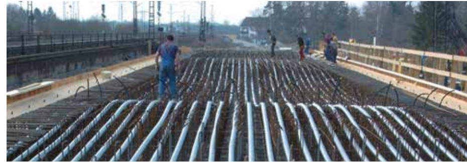
Bridge construction - channels for the strand
