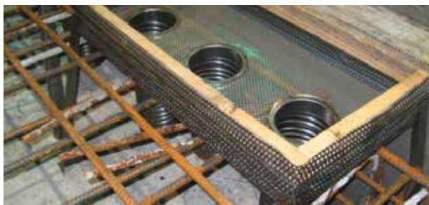
Formwork for machine foundation
